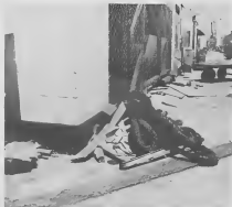
Another eye sore and unsafe situation: at Finger Pier # 2.
